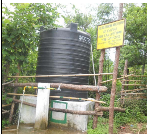
STORAGE TANK FOR DRINKING WATER SUPPLY
