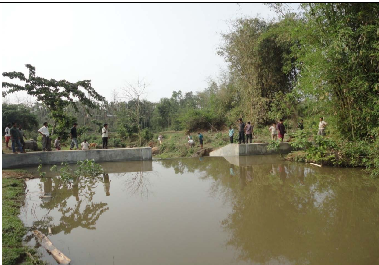
C. C. IRRIGATION DAM
