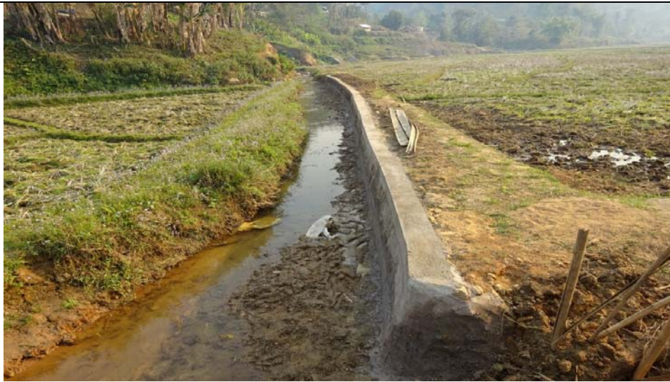
Protection Wall under RB-IWMP-VII in Ribhoi District
