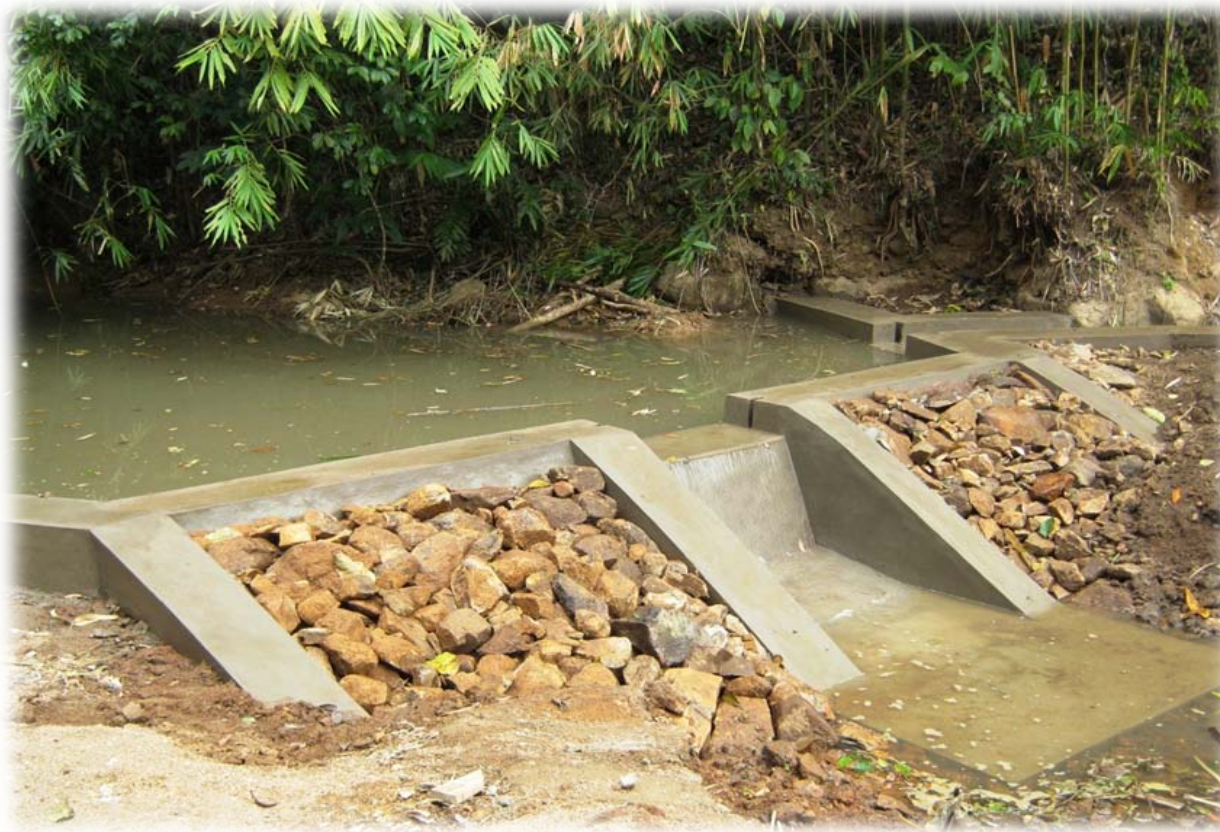
C. C. IRRIGATION DAM
